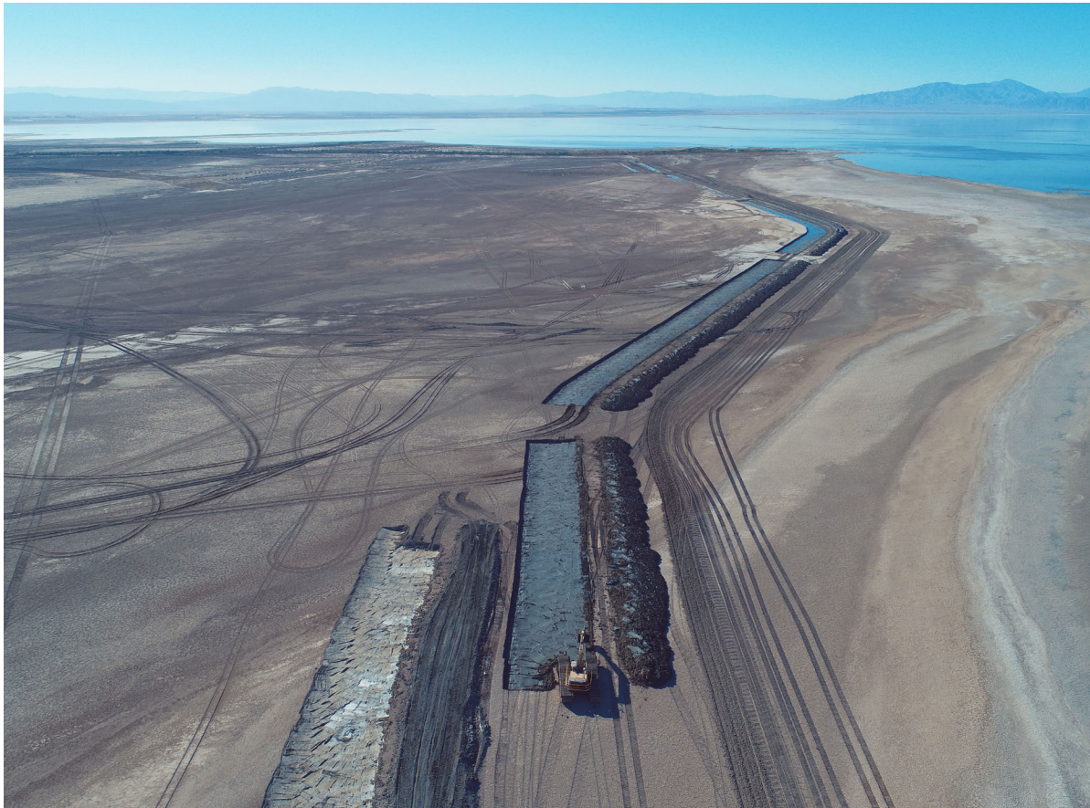
Construction at the SCH site: excavation of deep channel along northern berm of habitat pond.
