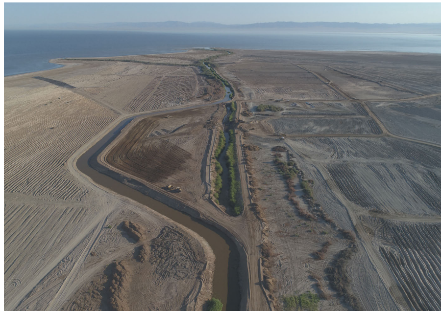
Figure 5. Construction of New River diversion to allow construction of the of intake structure for the SCH.
