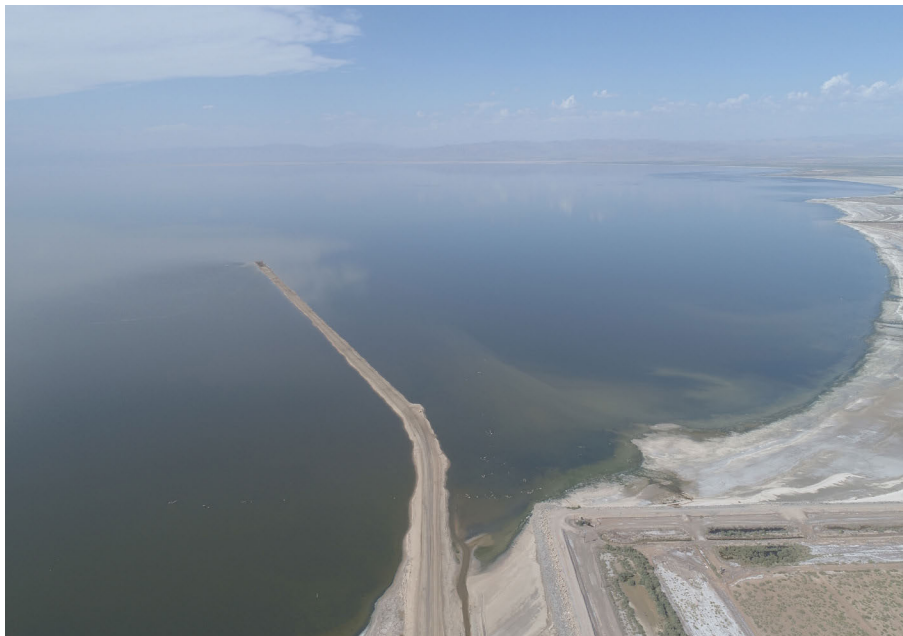
Figure 4. Aerial view of the completed causeway to the saline pump station, looking north toward the Salton Sea from the New River.
