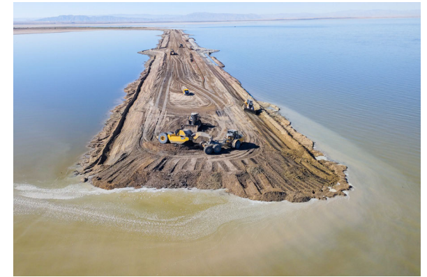
Figure 7. Riprap placement on the Sea-side of the SCH Expansion East Pond 1 berm.
