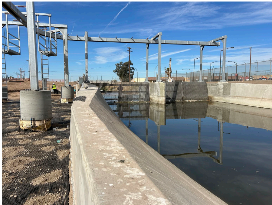
Figure 19. New River Improvement Project trash screen at the diversion structure on the New River.
