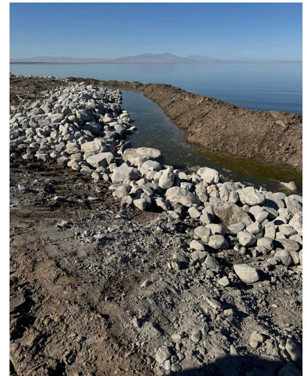
Figure 7. Riprap placement on the Sea-side of the SCH Expansion East Pond 1 berm.
