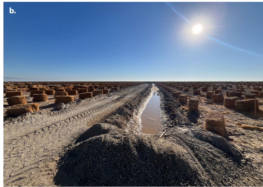
Figure 11. Site features and activities at the Tule Wash site. a) Seeding at Tule Wash D. b) Stormwater spreading furrow at Tule Wash B. c) Water tanks at Tule Wash A. d) Seeding at Tule Wash C.
